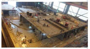
CB04A in final outfit position. P01s, paint and insulation underway
