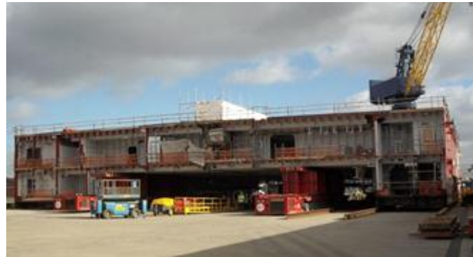
LK in place on the west quay.
