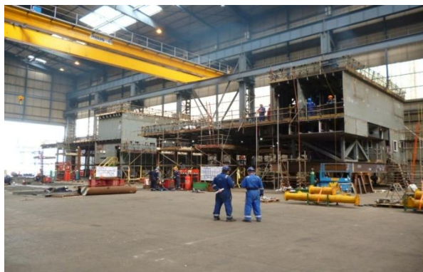
Ring J Port & Stbd units in build in construction hall.
