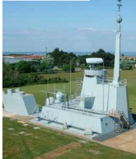
Mission System Integration Facility at Portsdown Hill
