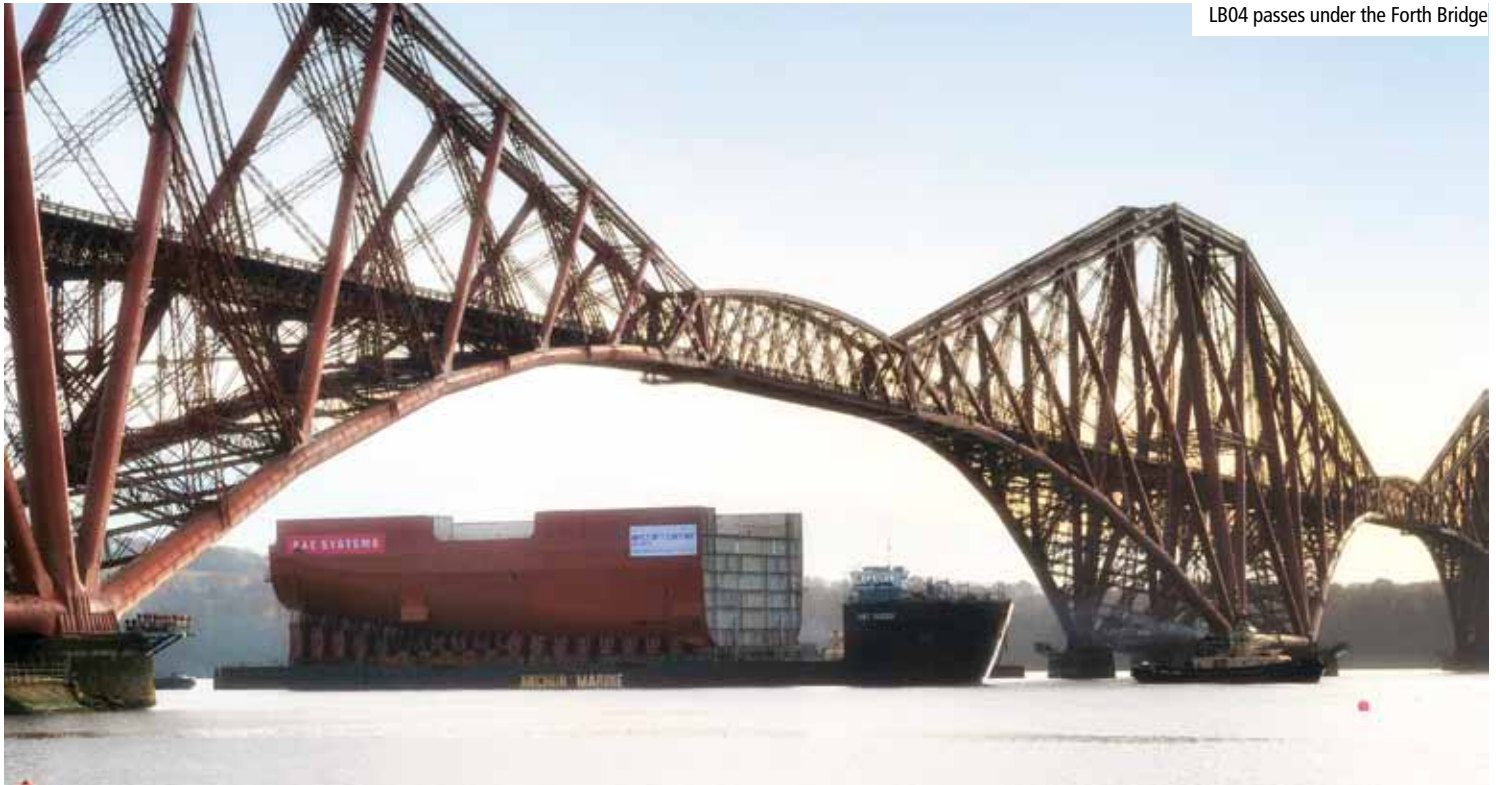
LB04 passes under the Forth Bridge
